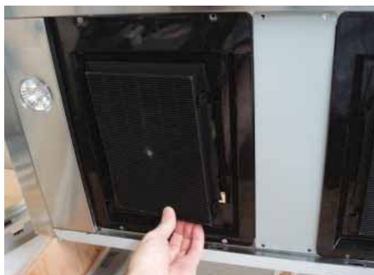
3. Install charcoal filters into charcoal filter brackets
