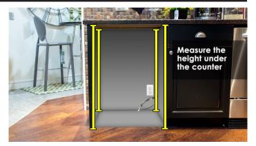
SIDE VIEW DISHWASHER Measure from the bottom of countertop to the floor in front of the dishwasher. NEWER FLOORING
