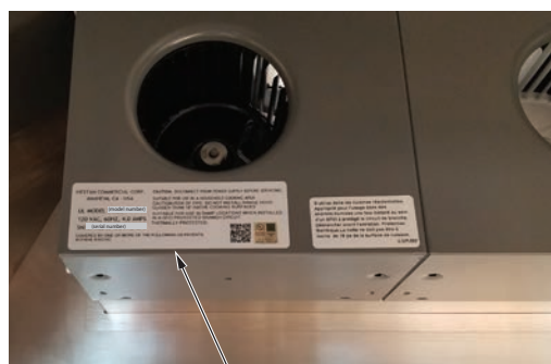
Rating label location
