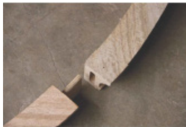
Mortise and tenon curved joints are laid out.
