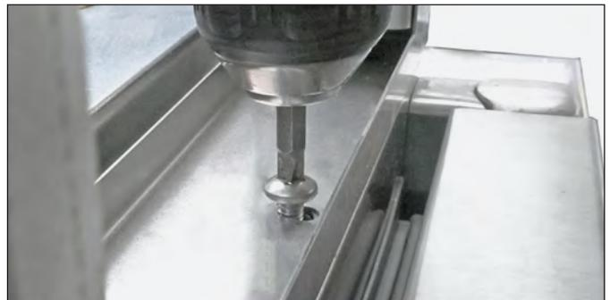
FIG. 10. Remove the screws from the metal channel.
